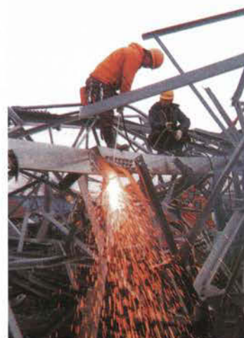
Cutting of steel tower fallen down 鉄塔倒壊
