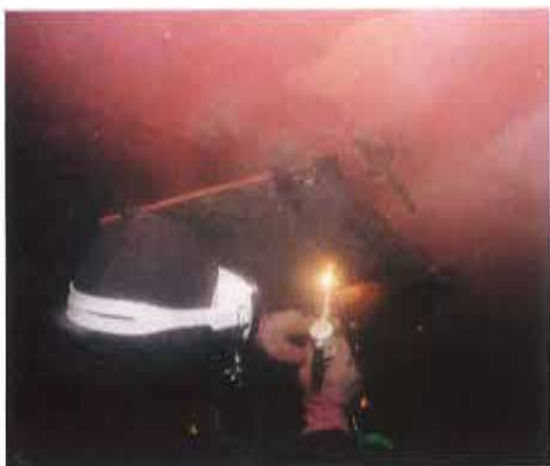
Under water cutting 水中切断
