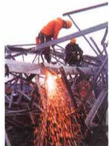
Cutting of steel tower fallen down 鉄塔倒壊
