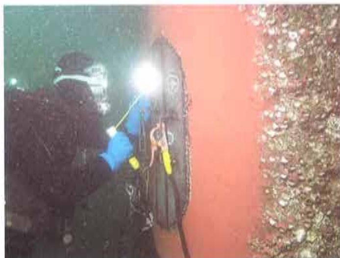
Under water welding 水中溶接
