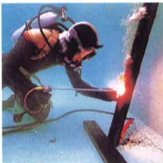
Under water cutting 水中切断
