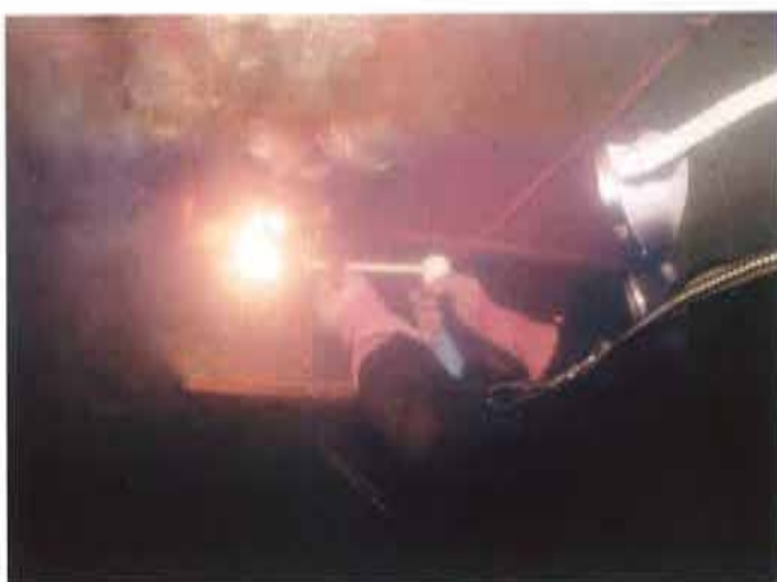
Under water cutting 水中切断
