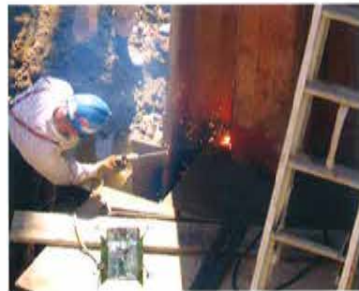
Cutting of sheet pile 鋼鉄板の切断
