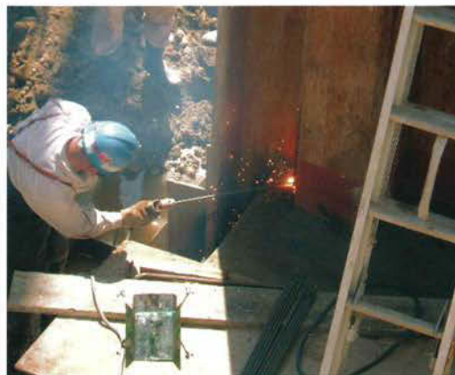
Cutting of sheet pile 鋼鉄板の切断
