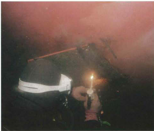
Under water cutting 水中切断
