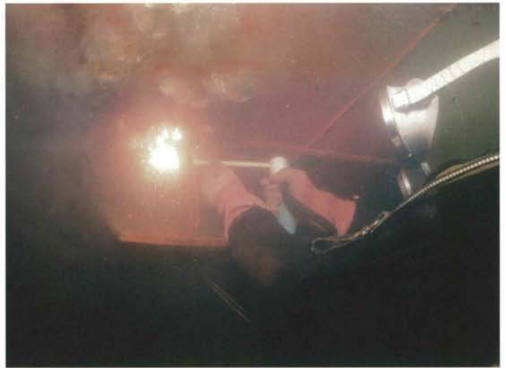
Under water cutting 水中切断
